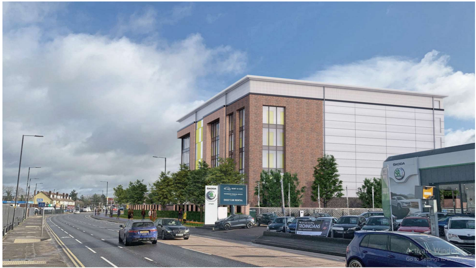
Figure 4 – View from the north west on Bath Road
